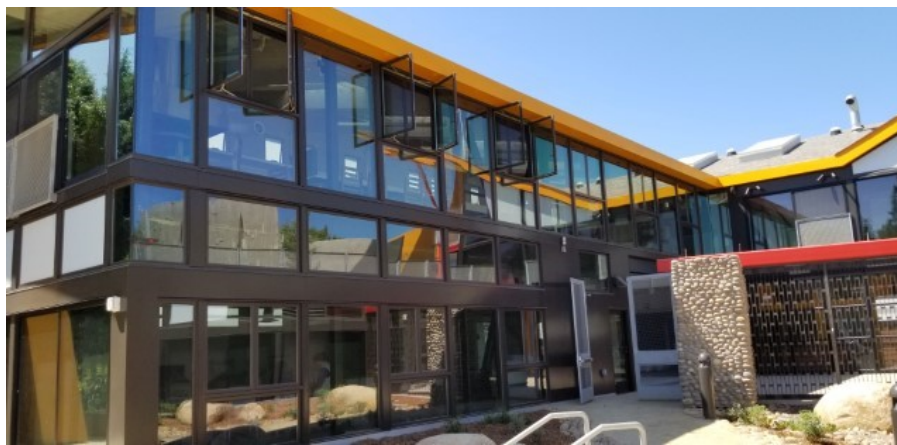
Main courtyard entrance
