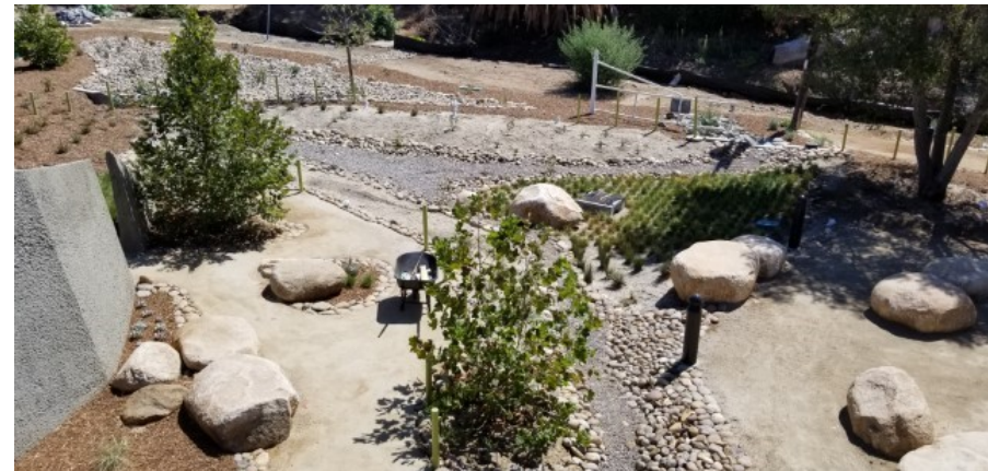
View of retention pond
