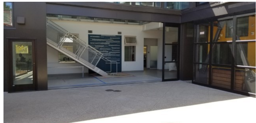
Main entrance large windows opened
